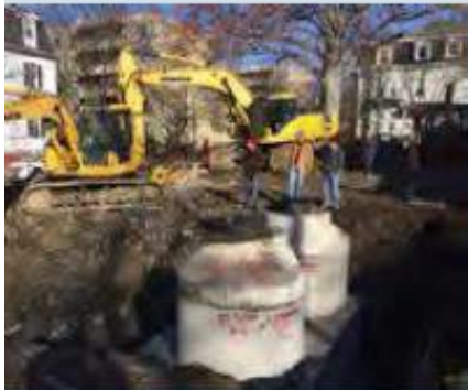
This page: Stormwater retention chambers were included in the redesign of both Symphony and Lincoln Park.
