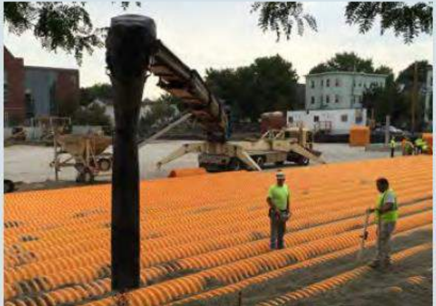
This page: Stormwater retention chambers were included in the redesign of both Symphony and Lincoln Park.
