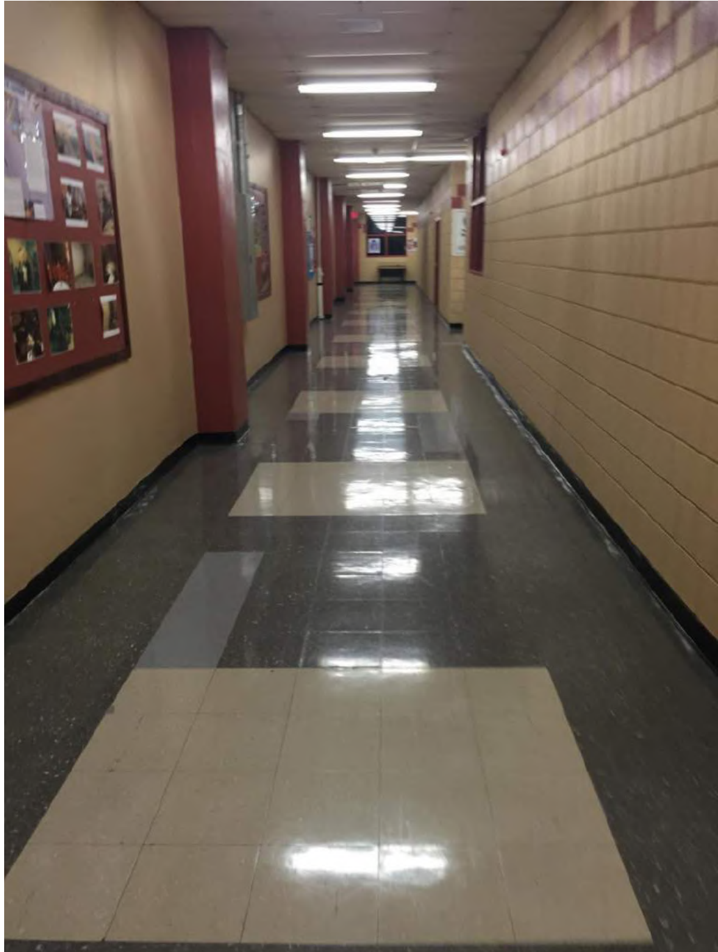
ACM Floor Tile in 1988 Wing
