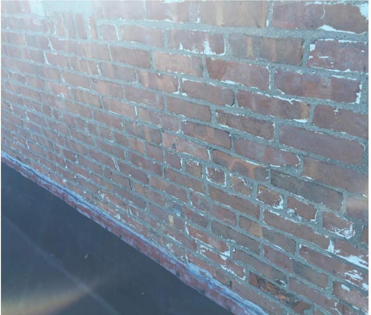
ACM Caulk on B Wing Roof Auditorium
