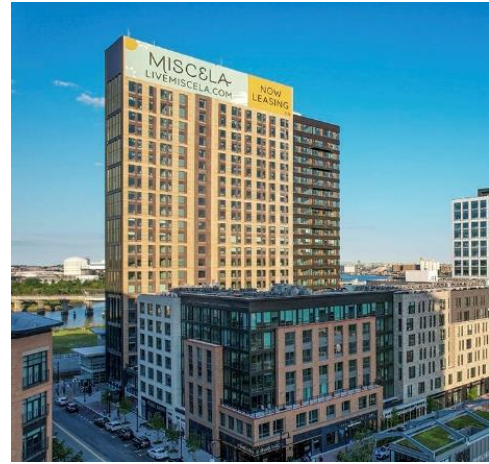
Figure 1: Miscela residential tower, which brought 500 new apartment units to Assembly Row, including 31 income-restricted units.
