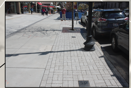
Precedent Image - City of Boston Conventional concrete sidewalk pitches to permeable paver strip with underdrains
