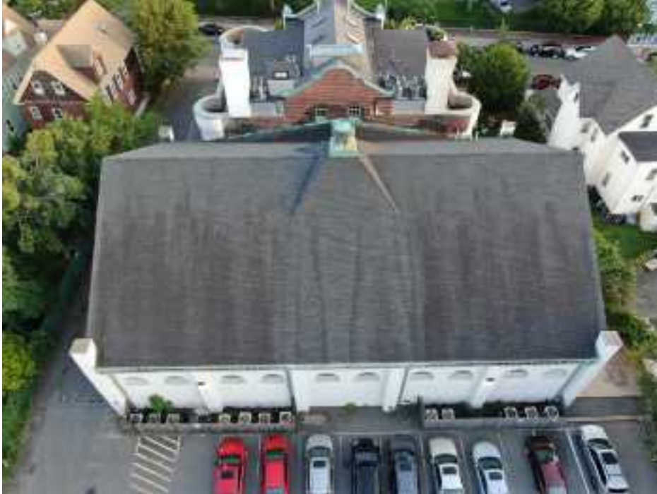
Figure 3. 191 Highland Avenue (Armory)
