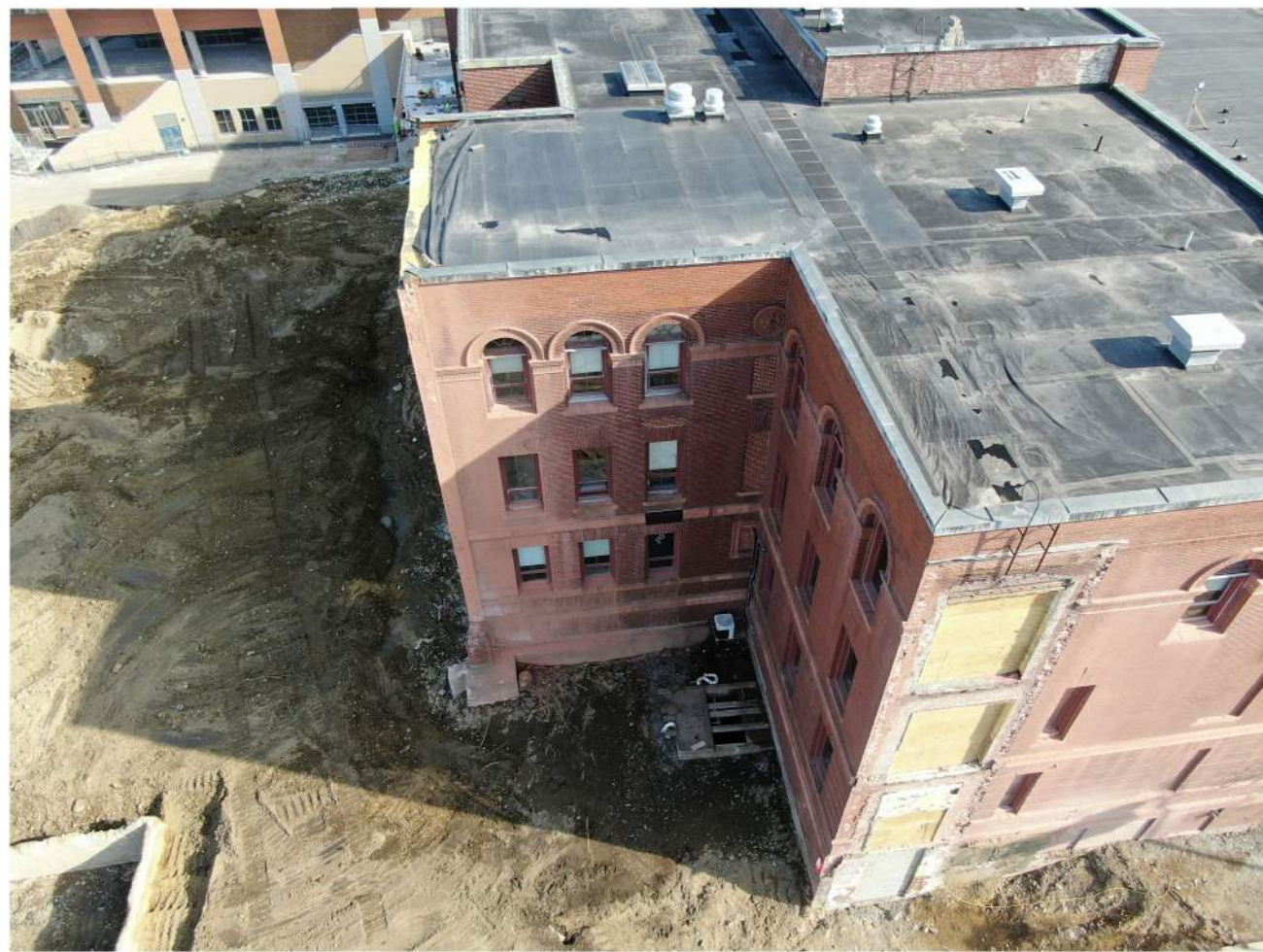
WEST ELEVATION DRONE PHOTOGRAPH
