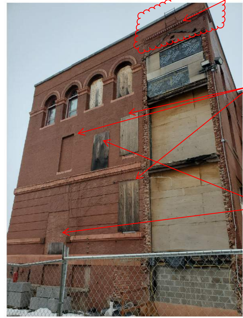
EAST ELEVATION PHOTOGRAPH
