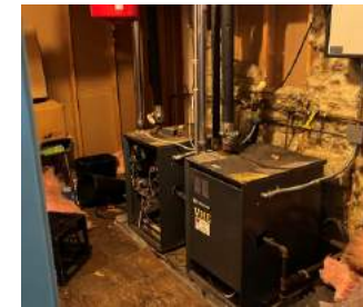
M4, M5. Abandoned gas-fired boilers on Third Floor, replaced with mini-splits
