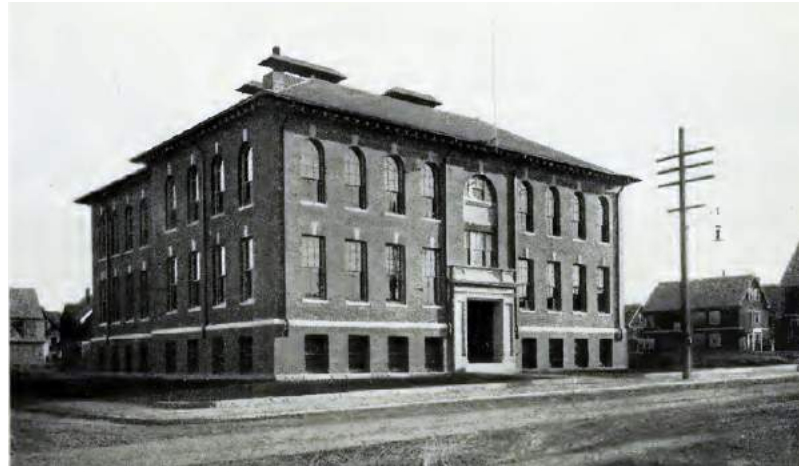
Photograph of the completed Brown School (predates the 1907 east expansion) Somerville School Committee Annual Report, 1901
