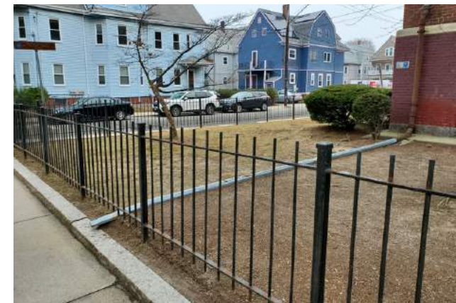
External downspouts daylighting to grade at the sidewalk
