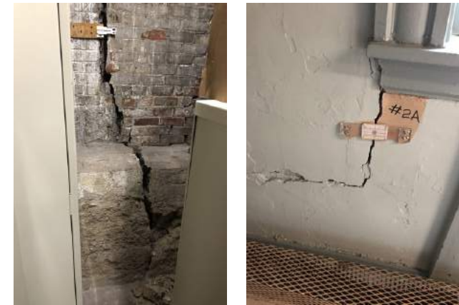
Interior view of wing interface; condition of interior finishes
