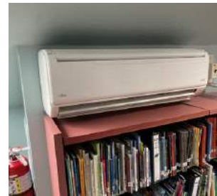
M4, M5. Abandoned gas-fired boilers on Third Floor, replaced with mini-splits
