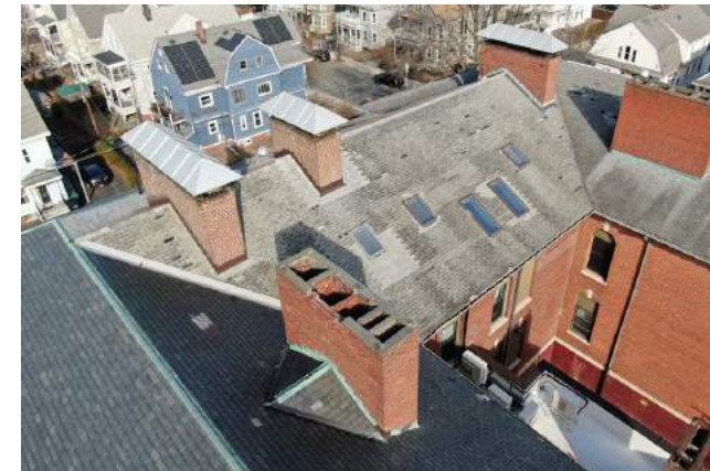
Drone photograph of Brown School roof
