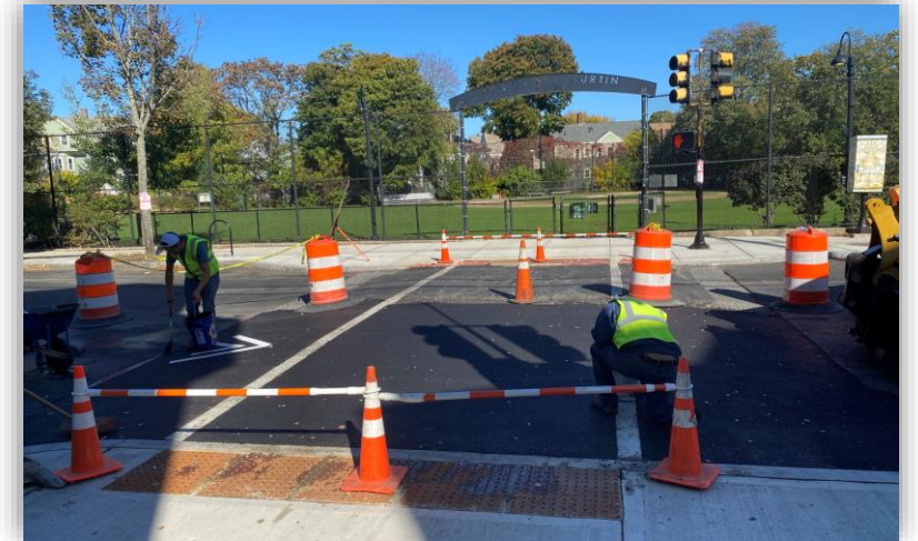
Raised crosswalk construction, October 2022
