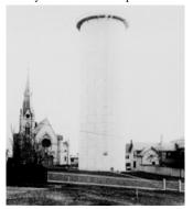
diameter and 100 feet high and estimated to hold about 530,000 gallons, was erected on top of Spring Hill, to provide suitable water pressure to the very highest lands in Somerville. Its water was supplied from a pumping station at the 'City Farm' (now housing the DPW), via Tufts Reservoir near Professor's Row, and ultimately from the Upper Mystic Lake .
