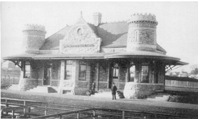
The West Somerville Station was built in 1888 as a stop on the Boston and Lowell Railroad. The station was demolished in 1934 and its granite stones were used to construct the Field House at Nathan Tufts Park as part of a Works Progress Administration (WPA) project.
